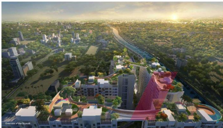
Overview of the Skywalk
